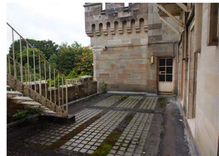
First Floor West Balcony
