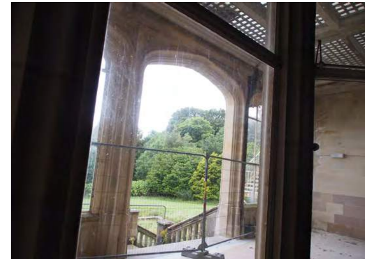
Covered west access from the Ballroom
