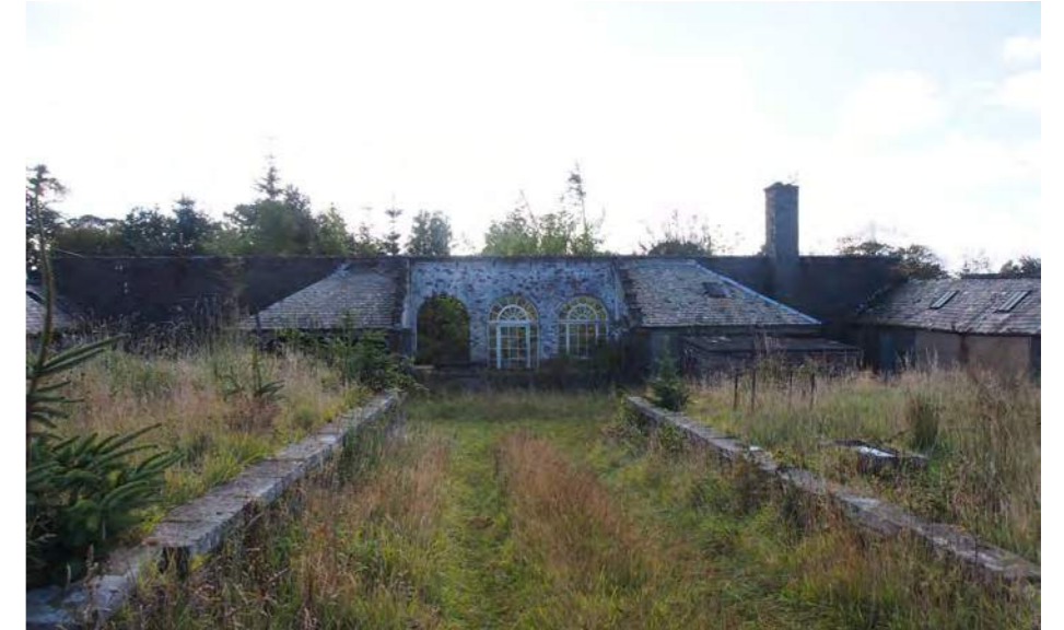
Greenhouse and workshop
